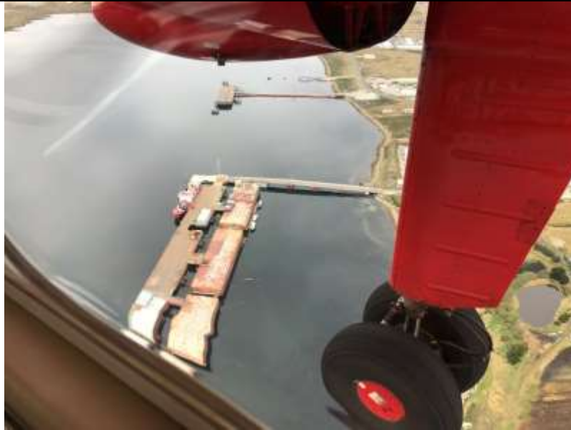
Figure 1 – A view of Stanley harbour from the FIGAS aircraft on a very calm day.
